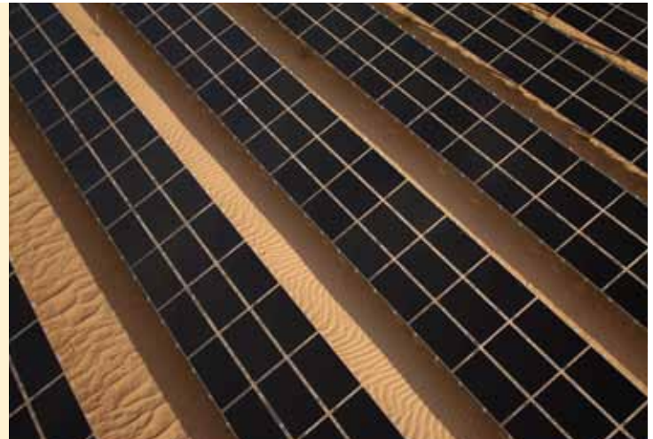
Solar photovoltaic panels at NRG's Blythe Solar Project.
